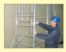
After opening the unit, serrated climbing rungs and diagonal braces are fitted.
