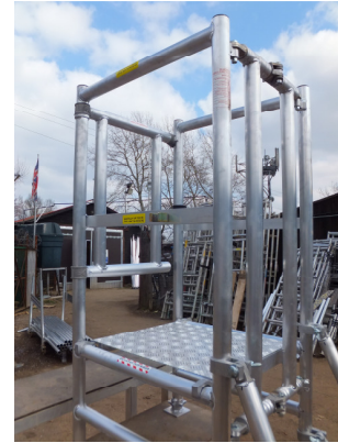
4. RELEASE PLATFORM FROM STRAP AND LOWER ON TO OPPOSING RUNG
