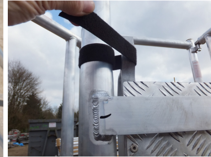
4. RELEASE PLATFORM FROM STRAP AND LOWER ON TO OPPOSING RUNG
